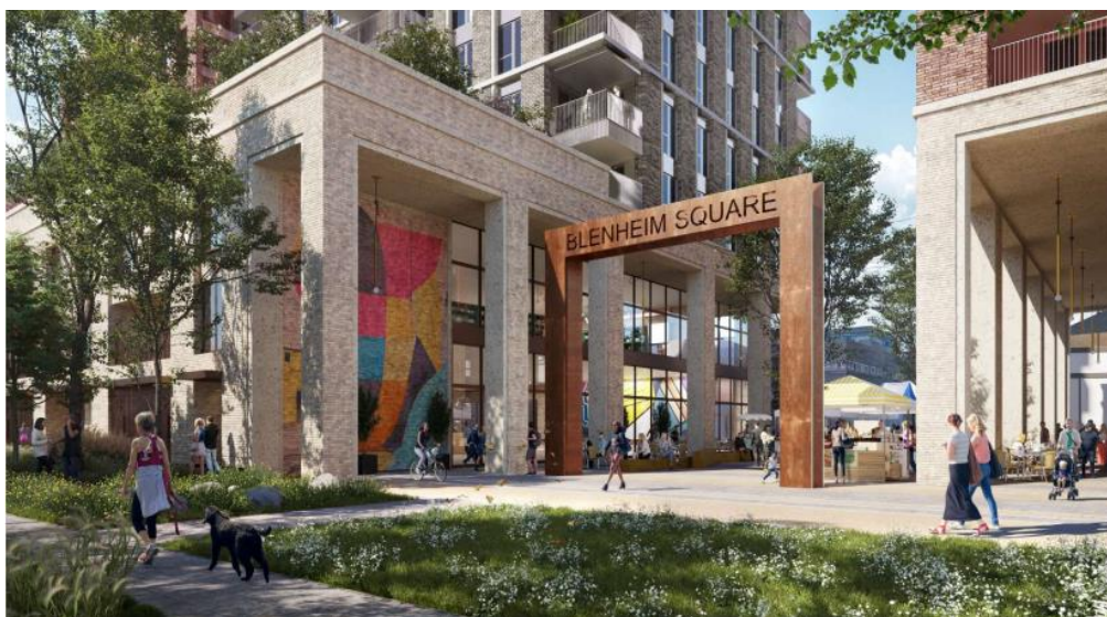
Fig. 2.3 View of Blenheim Square looking from Evelina Road (Planning Addendum Report).
